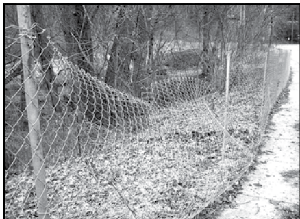
REPAIR OR REPLACEMENT NEED—SOON
