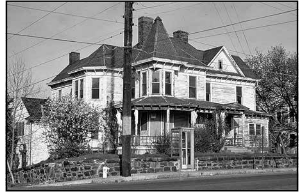
Gudger House in disrepair
