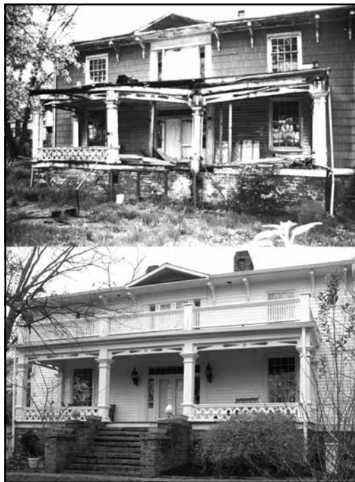
The Rankin House - before and after
