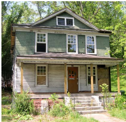
Baker House Flint Street - BEFORE
