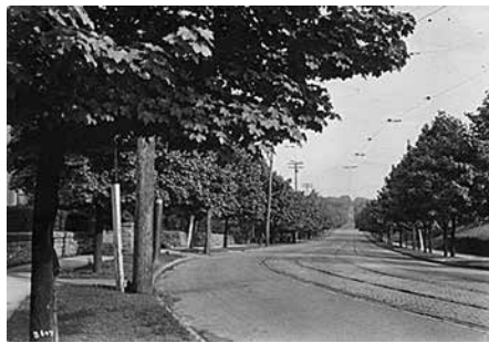
View long the side of Montford Avenue. Line of trees between the sidewalk and street on both sides. Street bricked and with two sets of streetcar tracks. Streetcar wires overhead. William Barnhill photo, circa 1920
