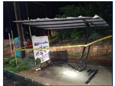
Montford’s designer bus shelter and historic panel destroyed in May.
